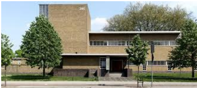
Servicebureau Ringbaan-Oost, Tilburg
